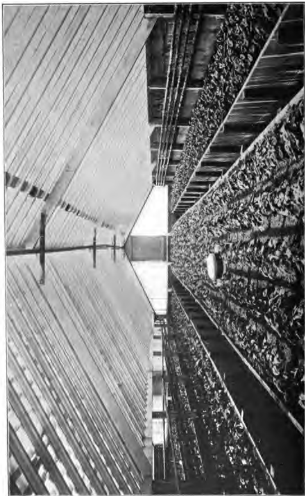
9.—Type of even span house, twelve feet wide, with two deep walks, showing heating pipes, and method of constructing beds, roofs, and ends.
